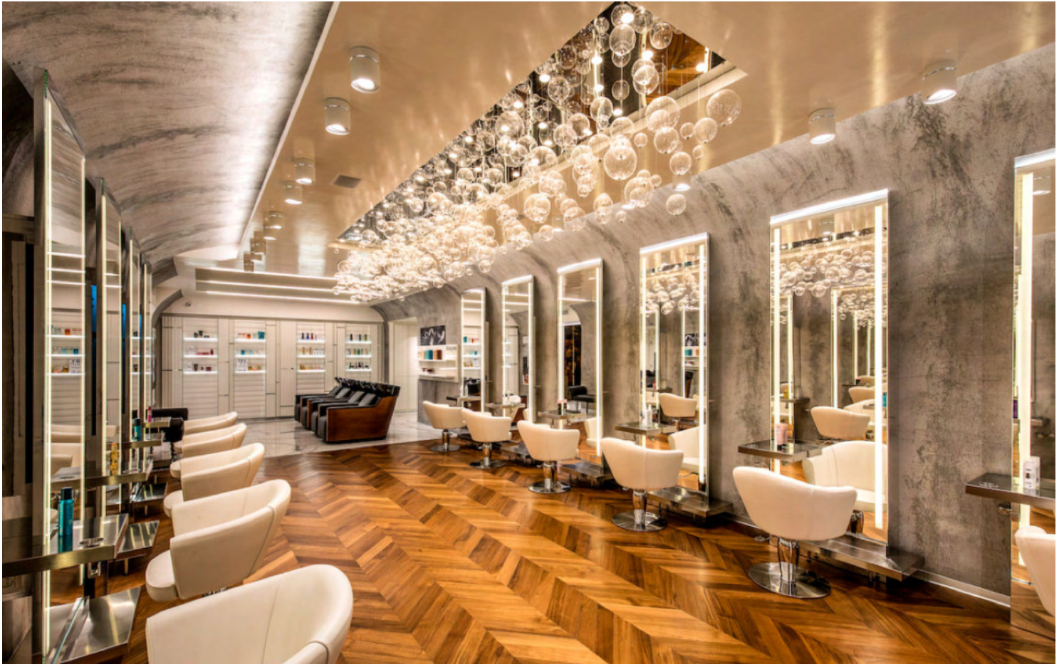
Custom Glass Installation - Beauty Salon Project
